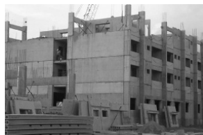
Hostel building at SRM University, Trichy Courtesy: VME Precast
