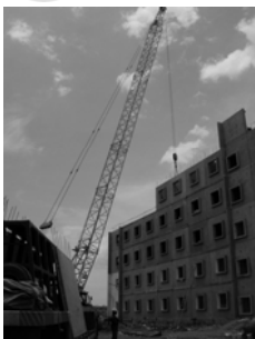
Hostel building at IIT Sri City Courtesy: Teemage Precast
