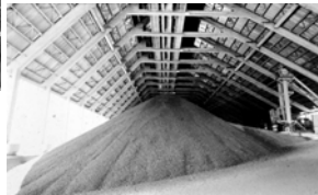
Material storage shed, Cement plant at Satna
