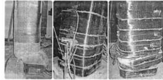
(a) Column RS-1 (b) Column RS-2 (c) Column RS-3
