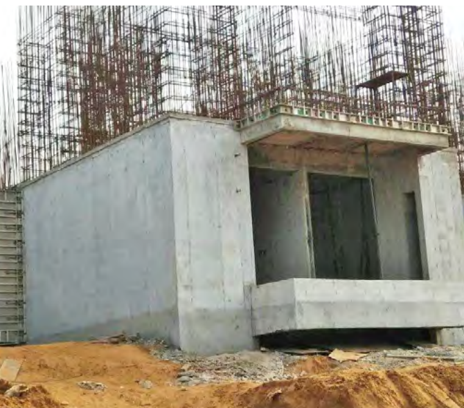
Monolithic Construction, CRPF, Kadarpur, Gurugram
